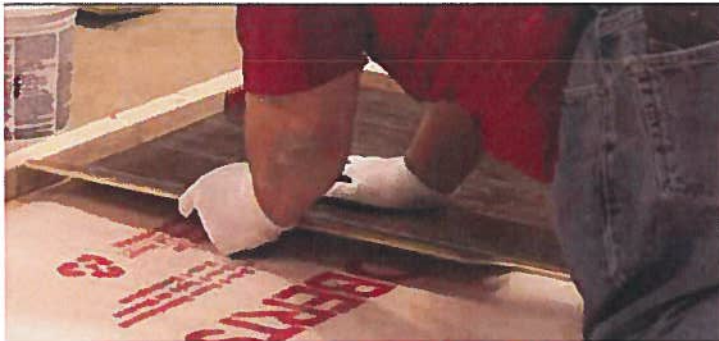
Tip: Wear gloves when working on knees and avoid tools that end in the palm of the hand.
