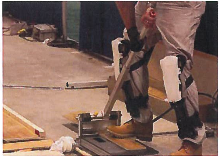
Tip: Use extended handles, work on raised surface (ie cut wood or laminates).
